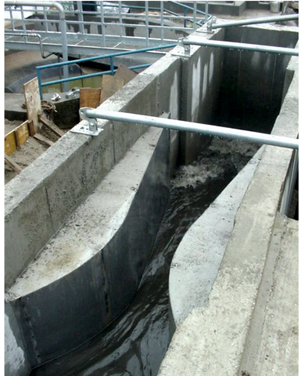
Concreted Parshall flume
