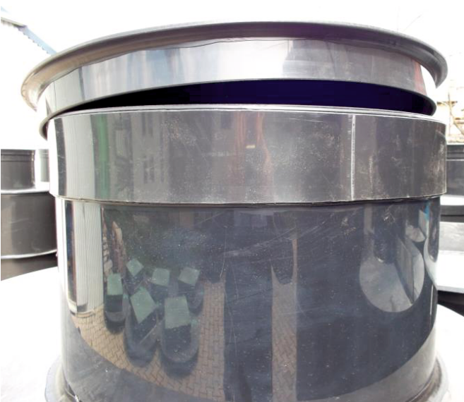
Entry „chimney“ on a water shaft
