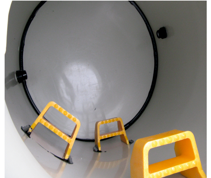
View inside - steps
